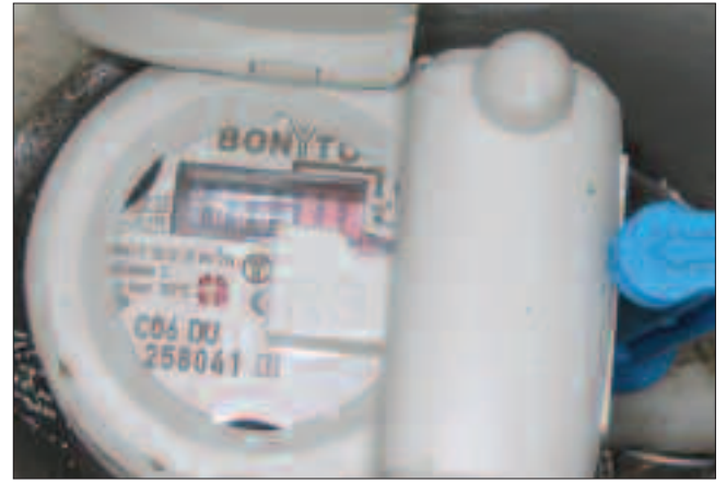
Fig. 2.13 Meter with attached transmitter located externally.
