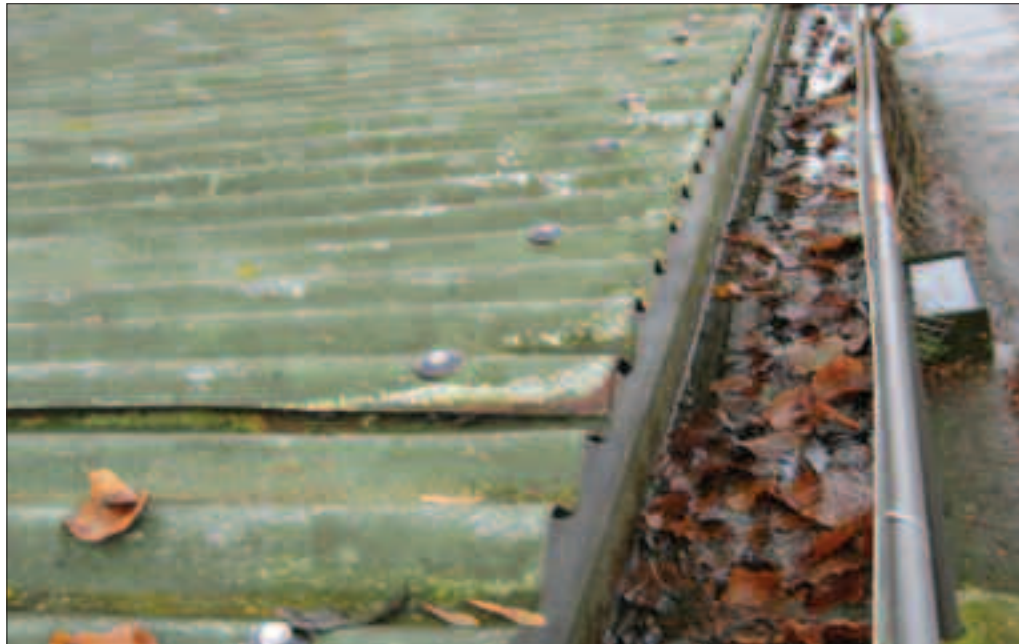
Fig. 3.10 Build up of leaves in gutter leading to failure of custom made filter.
