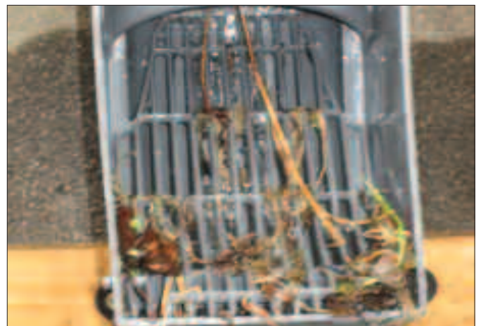
Fig. 3.13 and Fig. 3.14 A Lindab leafbeater TM and a BRAE TM filter installed.
