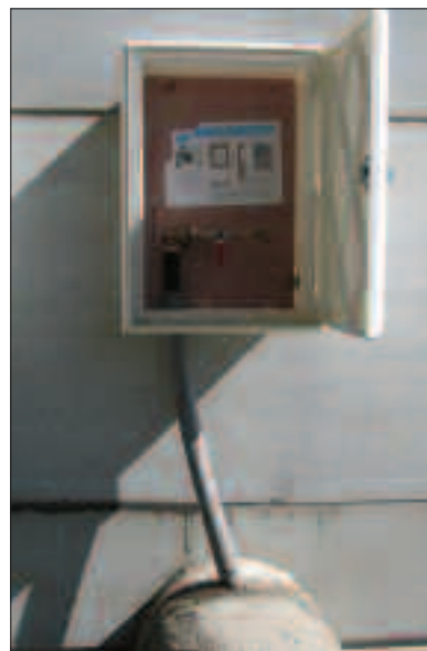
Fig. 3.8a&b Rainwater reservoir water quality sampling points.
