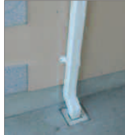
Fig. 2.7 Sealed downpipe to rainwater catchment system.
