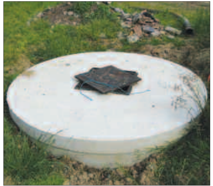
Fig. 3.3 Underground pumping tank.
