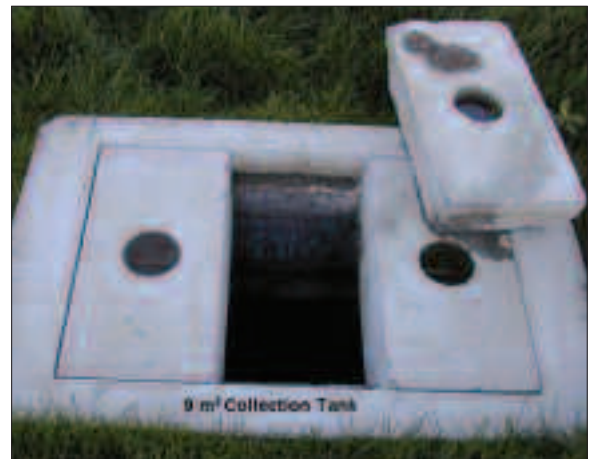
Fig. 2.3 Underground rainwater harvesting 9m³ storage tank.
