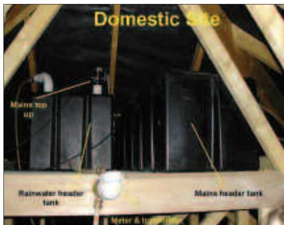
Fig. 2.2 Showing mains top-up to rainwater tank in attic.
