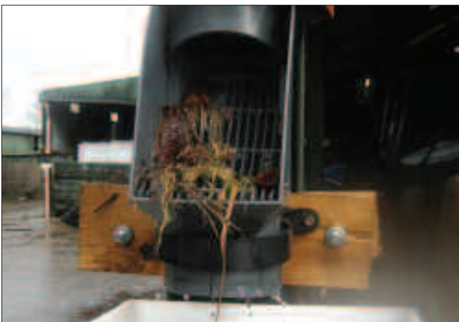
Fig. 3.13 and Fig. 3.14 A Lindab leafbeater TM and a BRAE TM filter installed.
